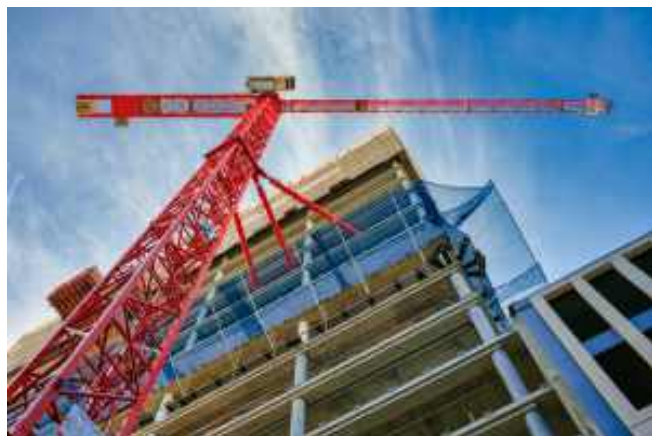
Picture Description: Personnel Safety Netting
